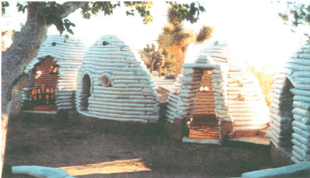
The Afghan "EcoDome" (top) and U.N. housing units use sandbags often filled with whatever is on the ground.
